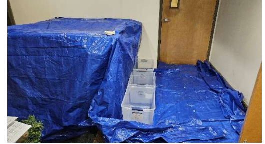
Winter weather exposes our historical building's many challenges.
